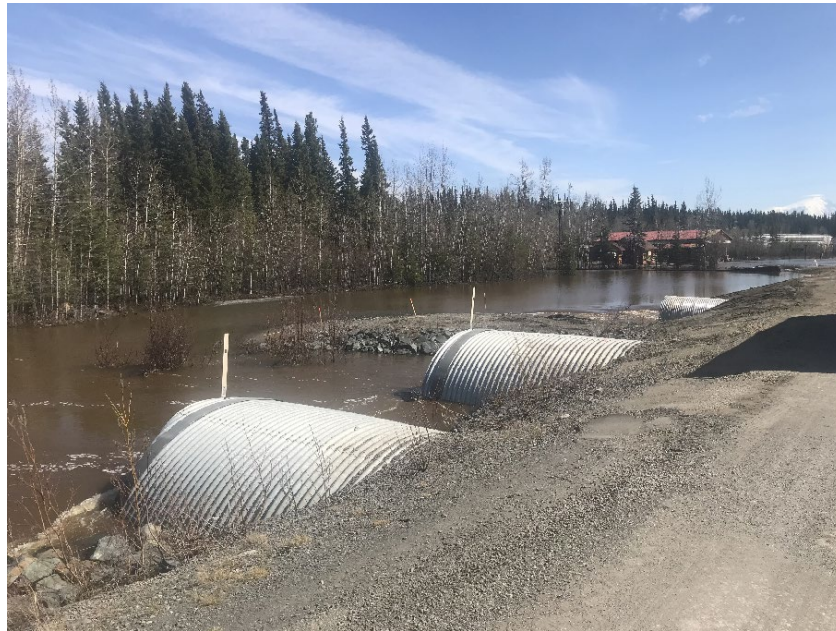
Glennallen, newly installed culverts, May 19, 2023
